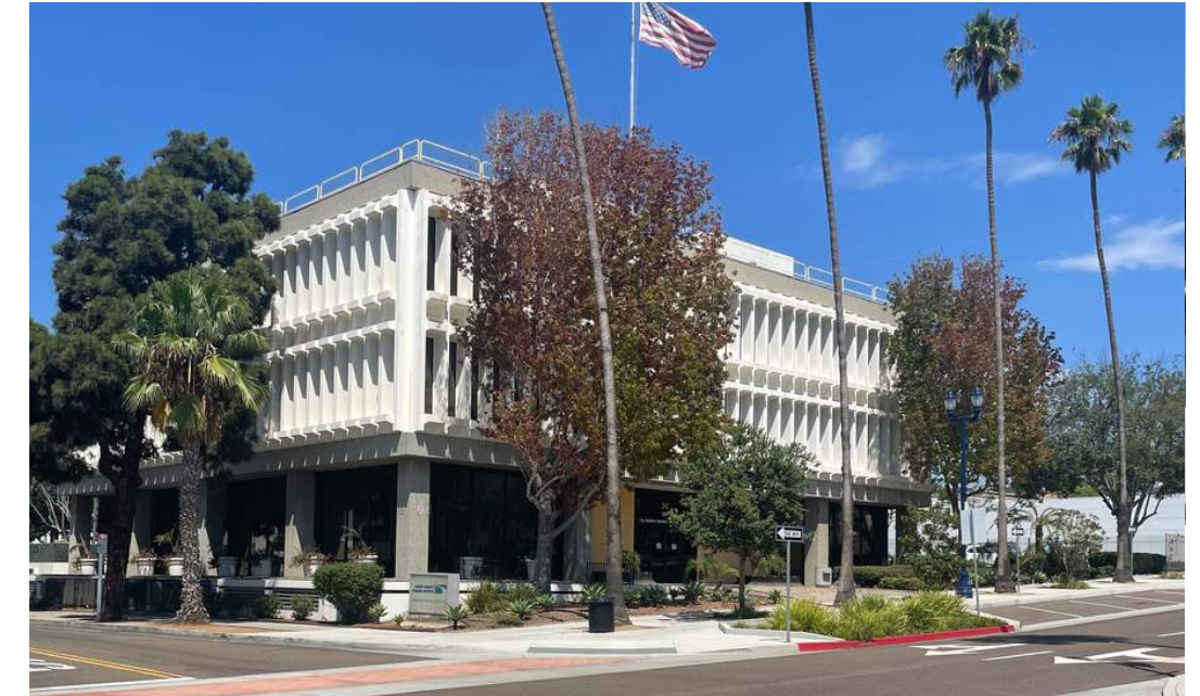
Existing Condition: 810 Mission Ave
