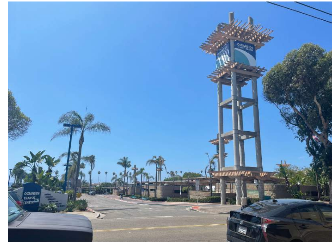
Existing Condition: OTC at 235 S. Tremont
