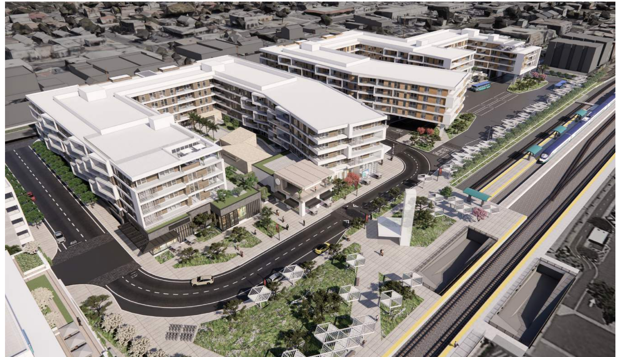
Station Plaza redesign in process.
