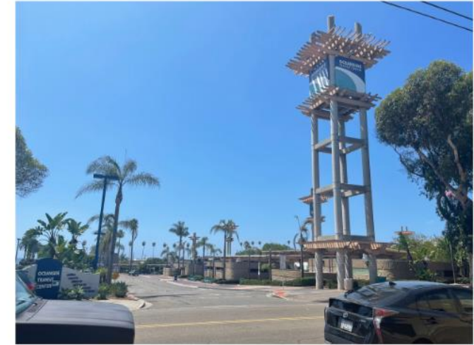
Existing Condition: OTC at 235 S. Tremont
